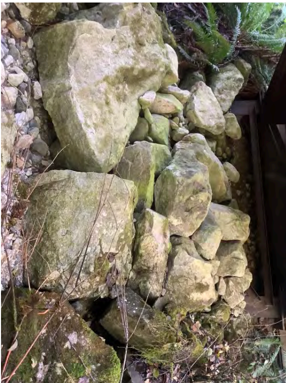
Right Bank Abutment when facing downstream
